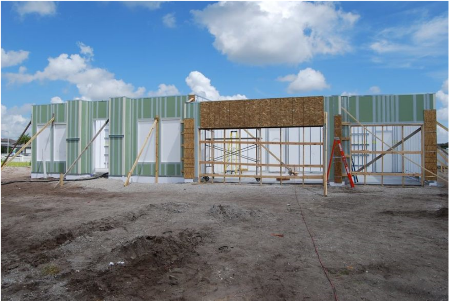
Meritage Homes Panelized construction techniques reduce labor demands.
